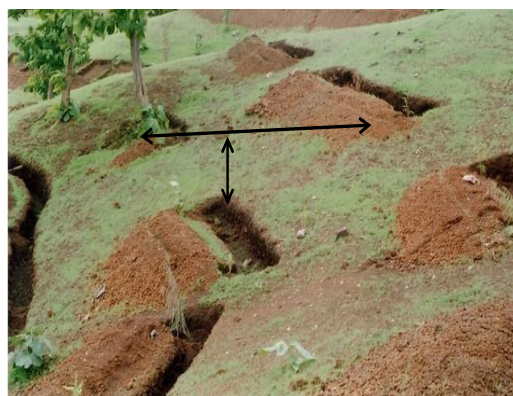
Figure 3. Staggered Contour Trench.
